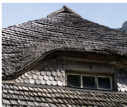
12.5 Wooden shingles of Picea abies on a roof appear gray due to the impact of acid rain.
