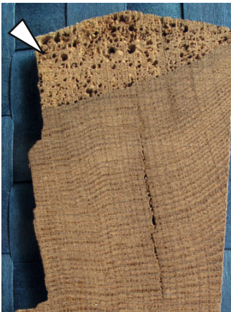
12.63 Heavily decayed sapwood of a beam of Quercus sp.
