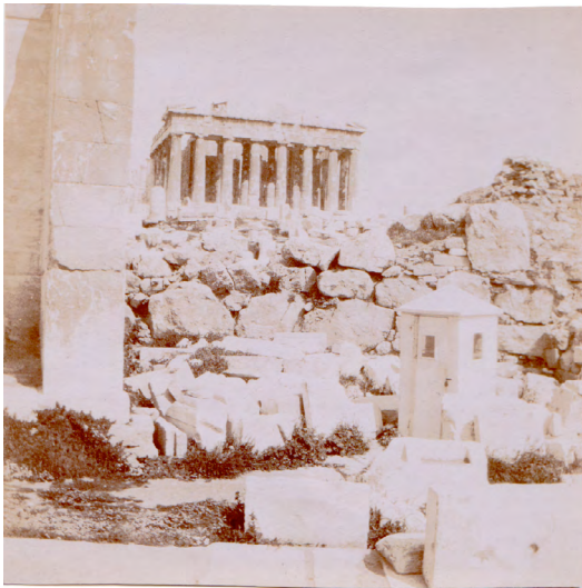
Figure 1.9. Remains of a wall at the entrance to the Acropolis. Amateur photograph, nineteenth or early twentieth century. 121
