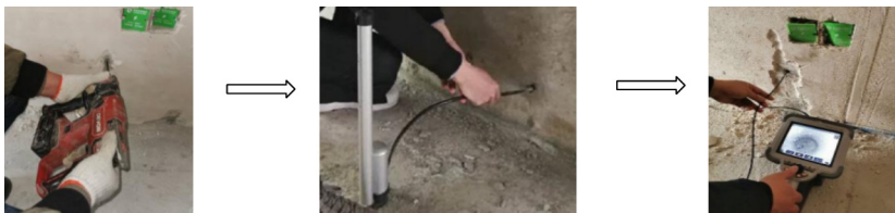
Fig. 4. Endoscopic method of grout hole drilling
