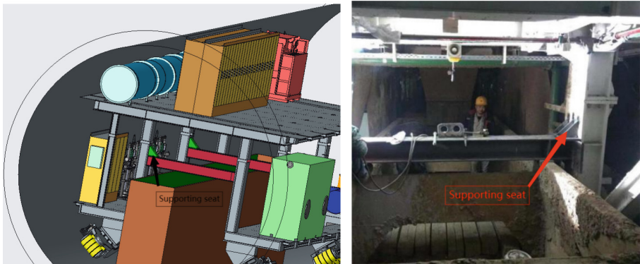
Fig. 11. Gantry supporting structure
