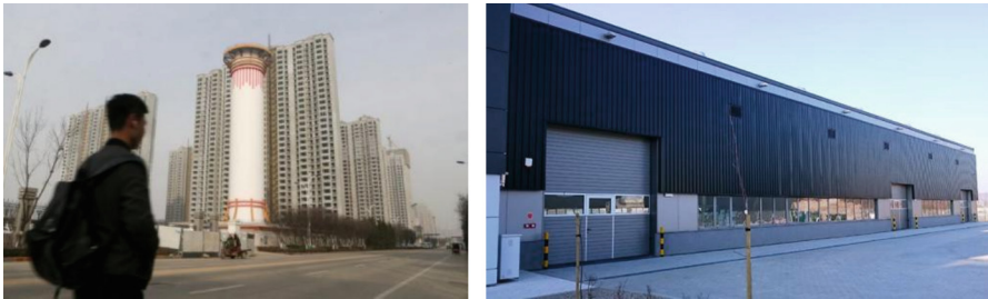
Fig. 1. Haze removal tower and solar collector wall.
