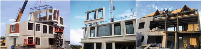
Fig. 3. Construction of prefabricated rural residential buildings.
