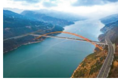
Fig. 6. Construction effect of Kui Zhou Yangtze River Bridge
