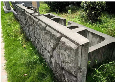
Fig. 1. Real-life photograph of the integrated assembly of prefabricated building panels and green modules
