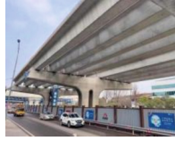
Fig. 5. Cantilever cover beam for Cha Wai Avenue
