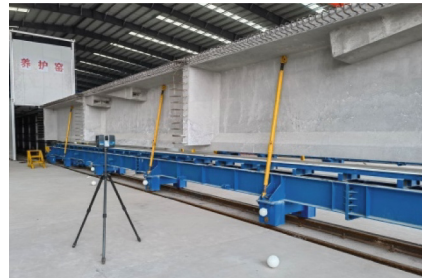
(b) Finished T-beam
