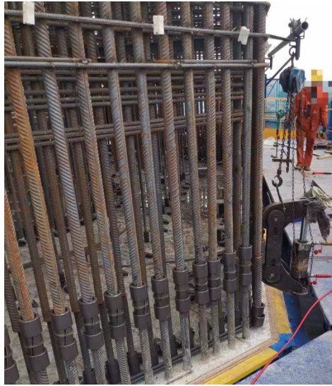
Fig. 7. Schematic diagram of the connection on the pylon of the reinforced bar product.
