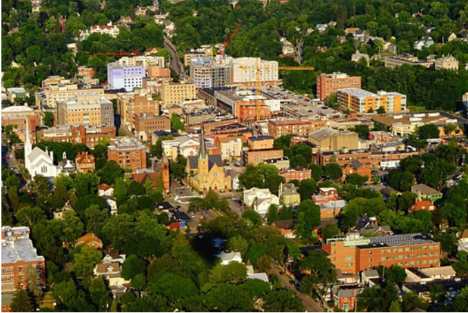
Fig. 2.2 A community consisting of interacting systems that provide the educational, environmental, public health, recreational, social, and transportation services people need and expect
