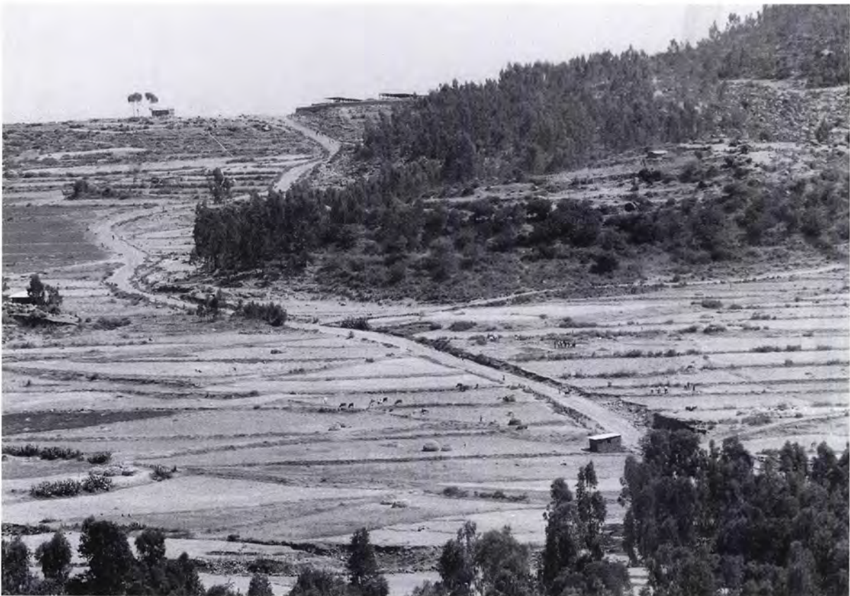
Fig. 236 View over D site from the south. The stone building right of centre houses the stone inscription discovered in 1981. D site is located in the cultivated fields immediately north of this building (cf. Fig. 237). The roofs visible on the horizon protect the Tombs of Kaleb and Gabra Maskal.
