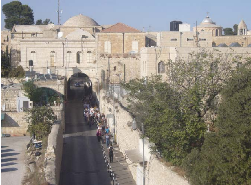
FIGURE 5.4 Jerusalem, buildings of the Armenian Patriarchate with the dome of the Church of St James to the right, from the city walls near the Sion Gate.
