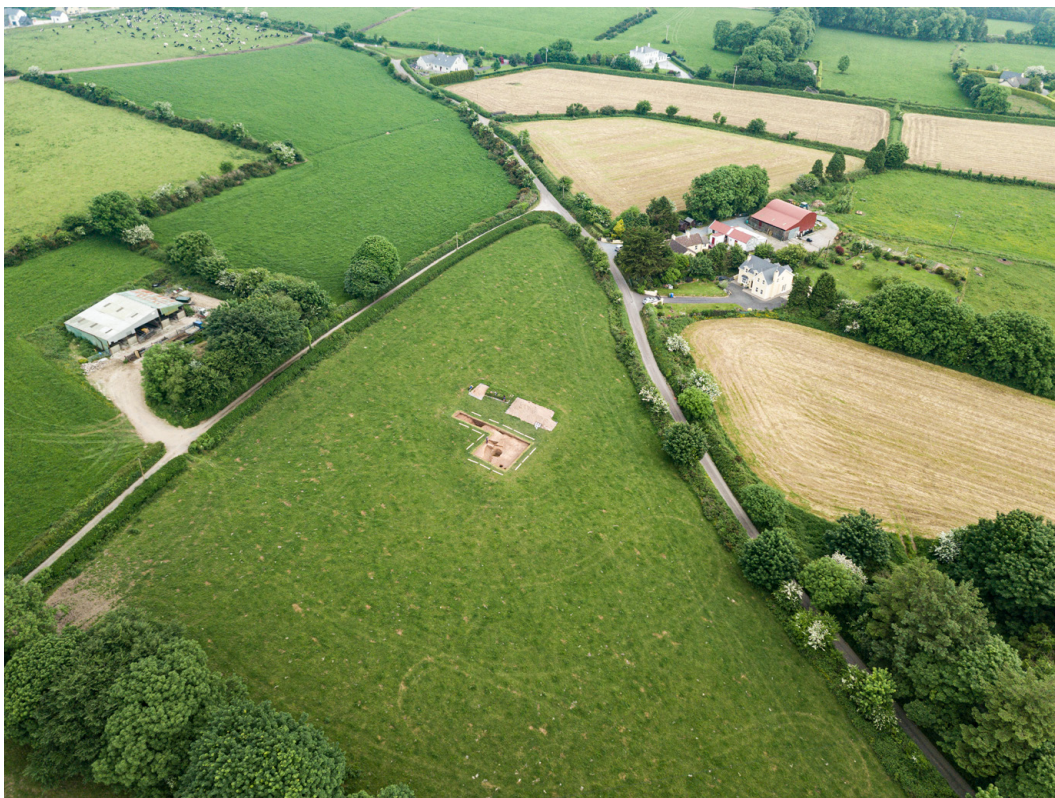
Figure 5.3 Aerial view of Lisheenagrine showing excavation area from south/south-west.
