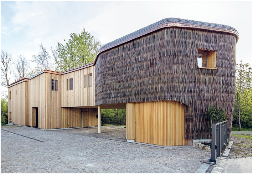
The rooms of this Ayurveda guesthouse in Rosenheim by Anna Heringer and Martin Rauch were composed with just a few primary materials: rammed earth walls, timber, clay casein floors, and handmade ceramic tiles.
