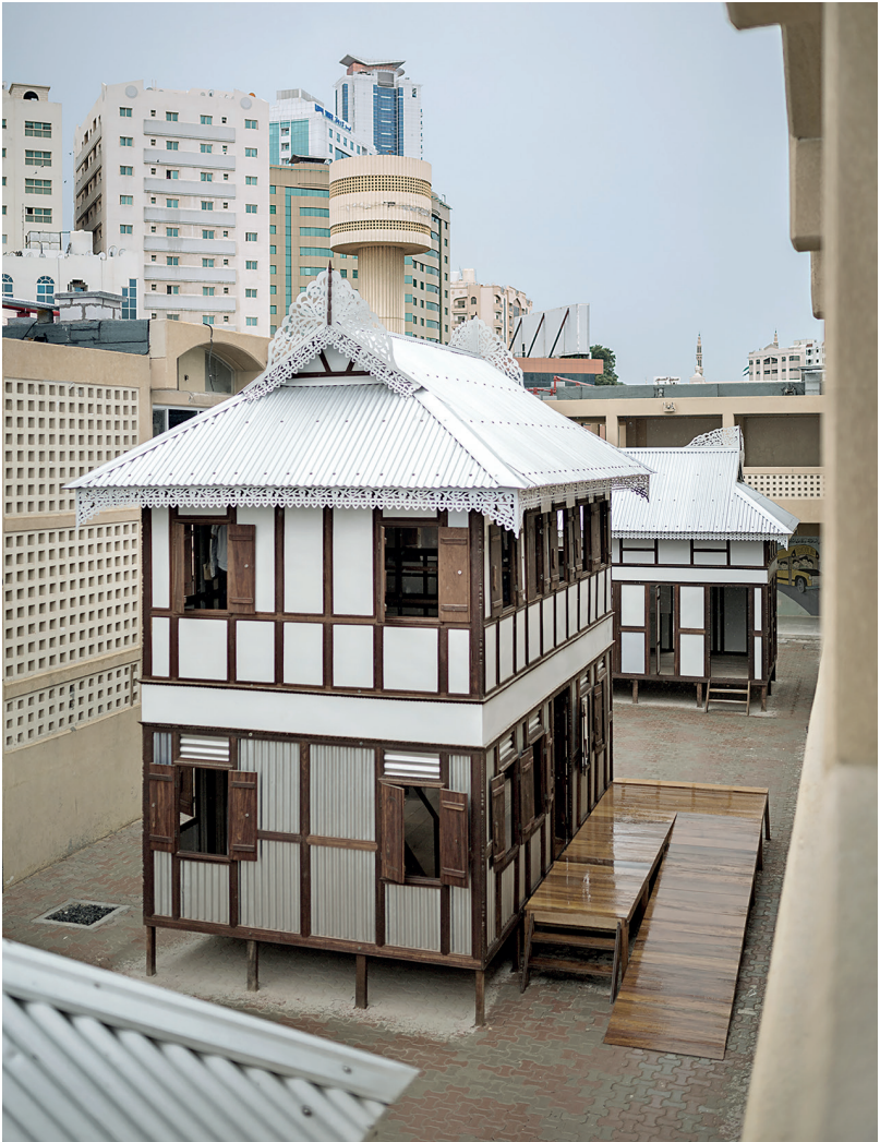
Vernacular construction: The timber frame structure of this typical prefabricated house, developed by residents of the Ganges-Brahmaputra river basin, is available for purchase at local markets in Lohajang, Munshiganj, and Dohar.
