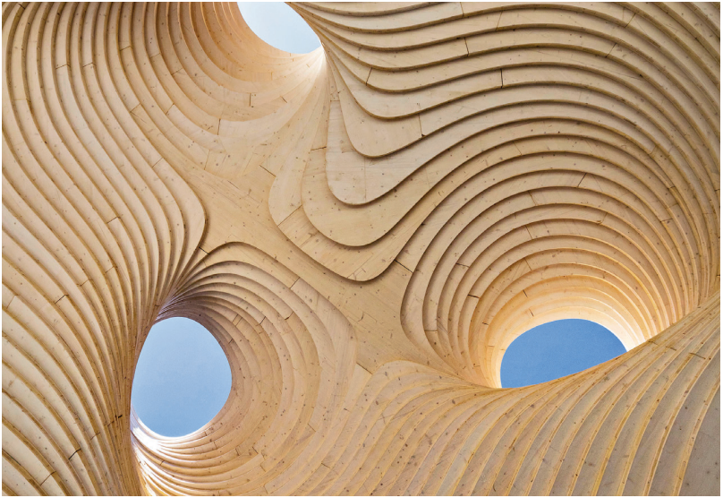
An impressive structure of conjoined timber domes was designed by Gray Organschi Architecture for their carousel pavilion at Mill River Park in Stamford, Connecticut.
