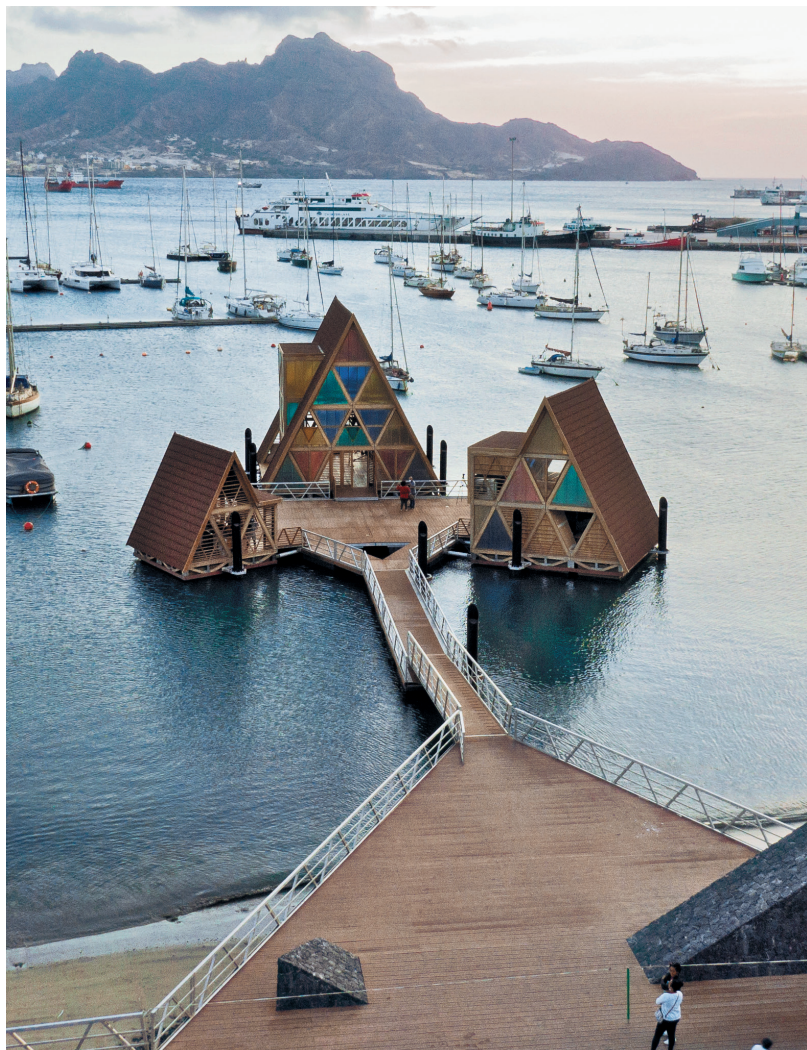
The Floating Music Hub by Kunlé Adeyemi is a space for music and cultural events made of prefabricated timber elements. It is anchored in Mindelo, Cape Verde.
