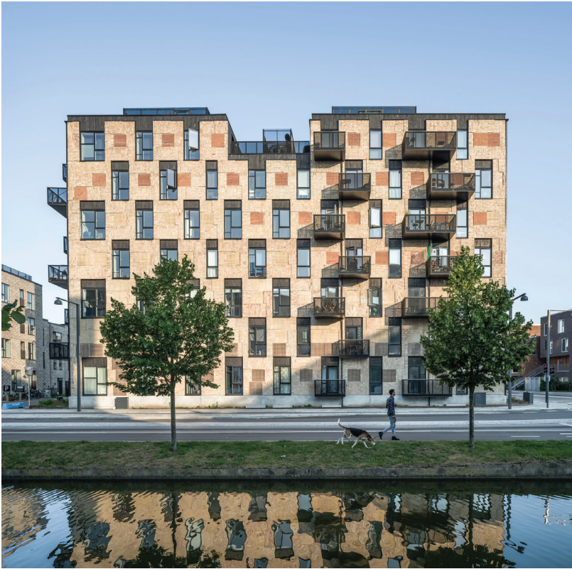
Resource Rows, a residential complex in the Ørestad neighbourhood of Copenhagen by Lendager Architects, features a patchwork facade of upcycled brick panels.
