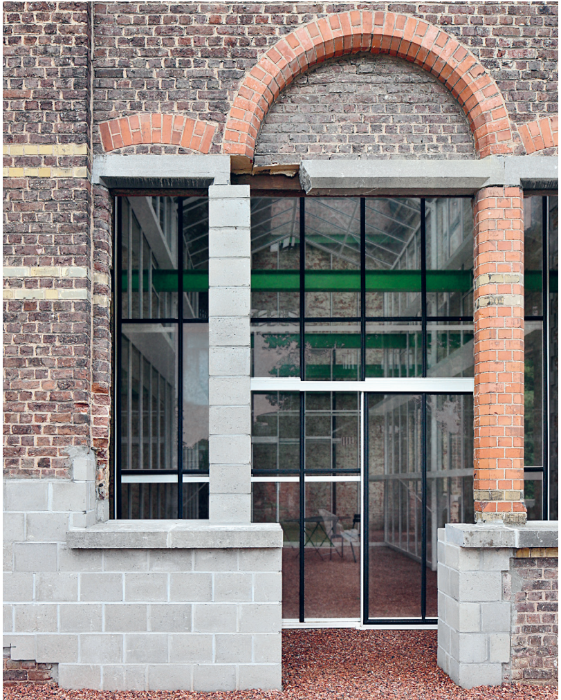
Manifesto for adaptive reuse: For the Caritas building in Melle, Belgium, Jan de Vylder, Inge Vinck und Jo Taillieu combined new concrete blocks with the historic brickwork.
