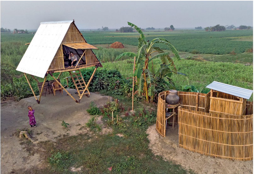
Khudi Bari (tiny house) are low-cost, mobile bamboo homes designed for resilience during flooding, by Marina Tabassum Architects.
