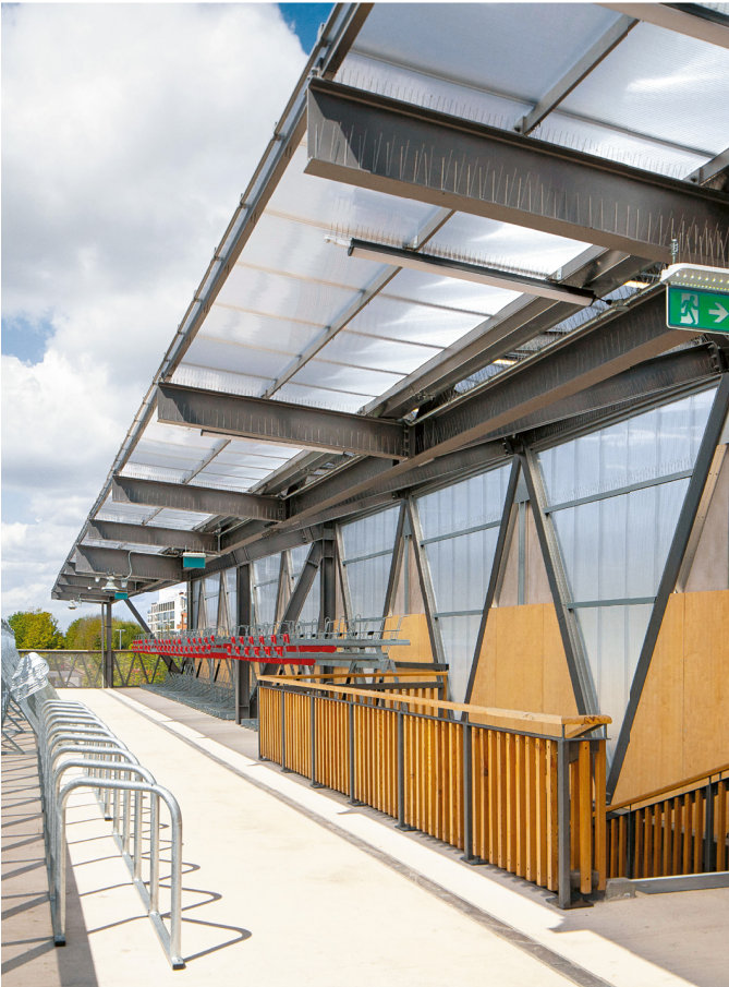
The Bike & Ride Station at Kingston Station in London features a three-story bicycle parking hub, a pedestrian bridge, and a recreational park along the train tracks.
