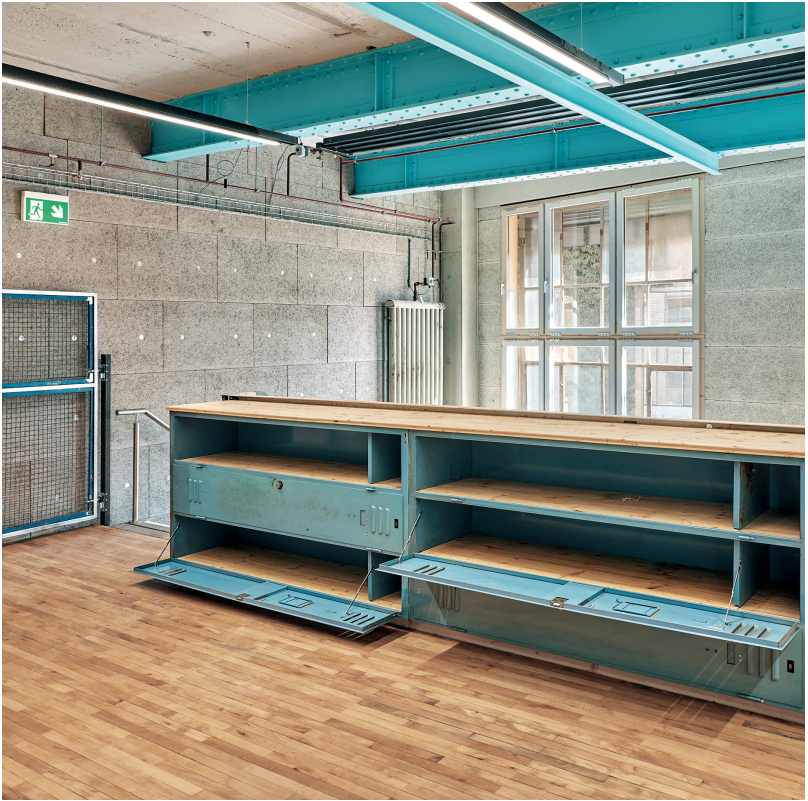
Old lockers now serve as safety barriers in the new K.118 workshop area.
