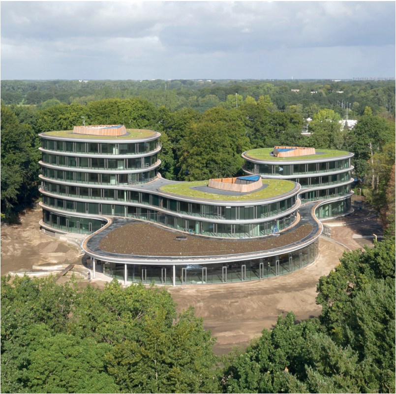
The Triodos Bank office building in Driebergen-Rijsenburg, designed by Rau Architecten, features a demountable wood-hybrid structure. All materials are recyclable and documented in a materials passport.
