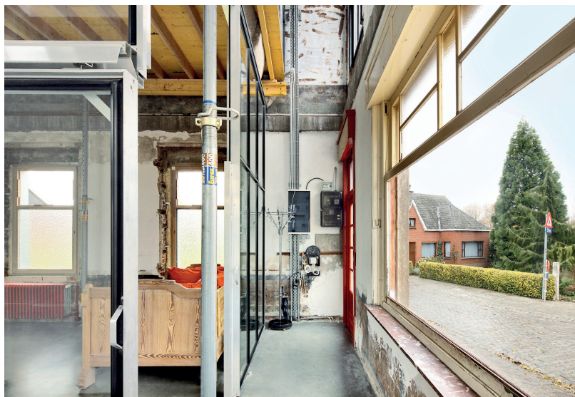
Living bricolage: Formerly a café, the Rot-Elle-Berg house near Ghent was renovated in 2013 by De Vylder Vinck Taillieu into a private residence. Construction scaffolding and concrete formwork were integrated as permanent elements within the interior.
