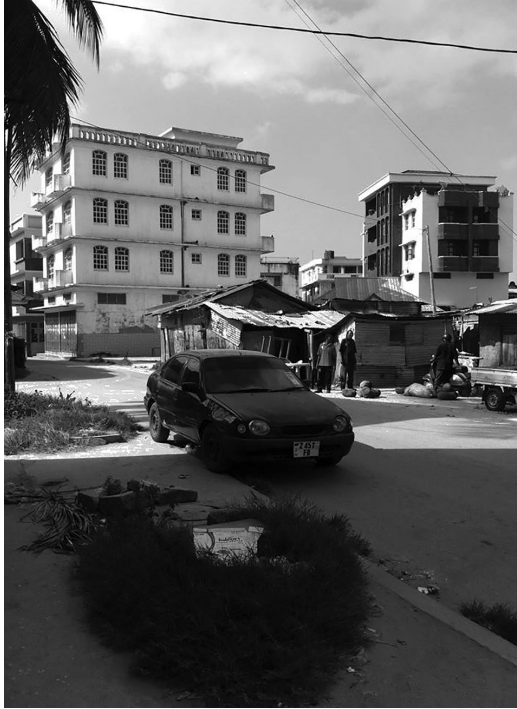
Figure 12.5 New Multi-Story Apartments, Kikwajuni, Zanzibar, January 2017. Source: Garth Myers.
