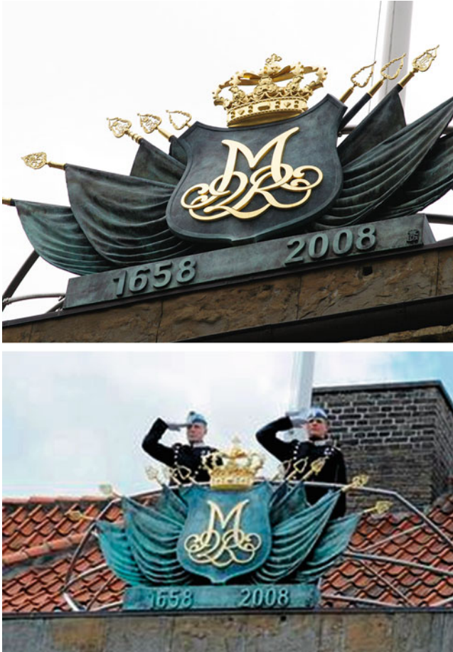
Figs. 1 and 2 The cartouche on the roof of the Rosenborg barracks, in two different stages of patination (Fig. 1 copyright Evelyn Iversen)
