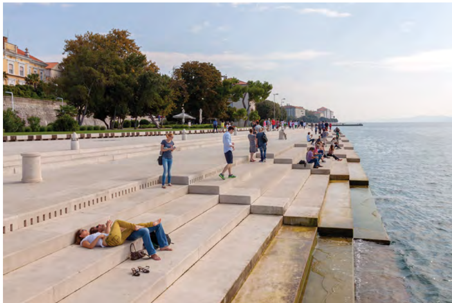
Figure 12.26 A view of the Sea Organ showing the steps and the holes along the top step where the sound emerges (Source: Creative Commons Attribution-Share Alike 2.0 Generic Licence)
