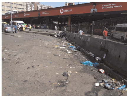
Figure 2. A portion of the stations turned into a dumping site.
