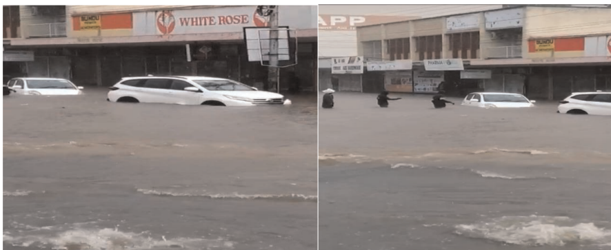
Figure 1. Showing the flooded road due to inadequate drainage system.
