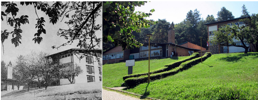
Figure 2. United Nations Refugee centre in Banja Koviljača. Architect Mihajlo Mitrović, 1964, a) in 1966 (source: Mihajlo Mitrović: izložba arhitekture, Muzej primenjene umetnosti Beograd, 13-25. april 1971 ), and b) in 2018 (source: http://arhiva.kirs.gov.rs/docs/azil/Centar_zazil_Banja_Koviljaca.pdf ).
