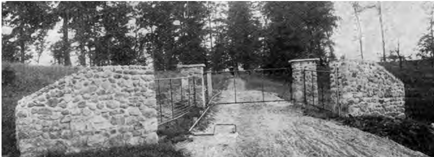
The entrance lane to Virginia Meredith's Norborough Farm in Cambridge City, Ind. The device in the lane would automatically unlock the gate when her carriage crossed over it. Reproduced from Dignam's Magazine .
