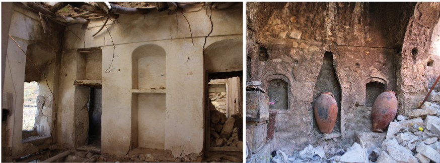
Fig. 4. Doors and windows transformed to wall niches used as shelves, cupboards or fire places.
