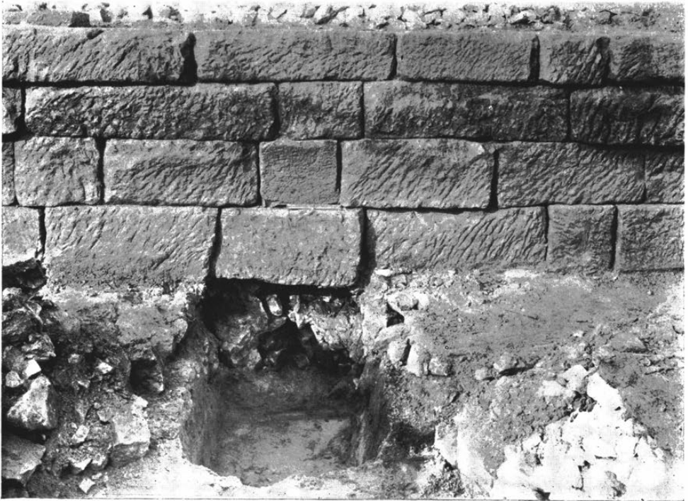
Fig. 2. East wall of Podium showing clay and stone foundation
