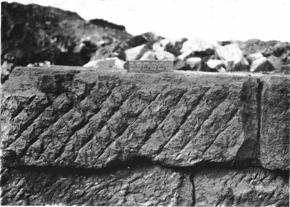
Fig. 2. Diamond broaching of stone in east wall of Podium
