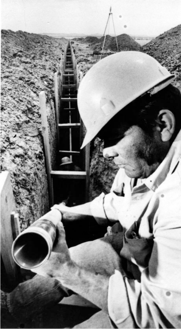
Fig. 7.6 The TE_{01} mode circular waveguide was buried alongside the railway track to transfer the local oscillator and IF signals between the central control building and each antenna. Credit: NRAO/AUI/NSF
