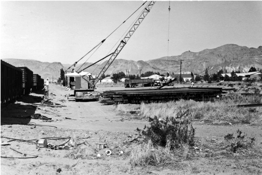
Fig. 7.9 Unloading surplus rail in Socorro. Crane is unloading Crab Orchard rail from rail cars. The truck in the background is leaving with rail for the VLA site. Credit: NRAO/AUI/NSF
