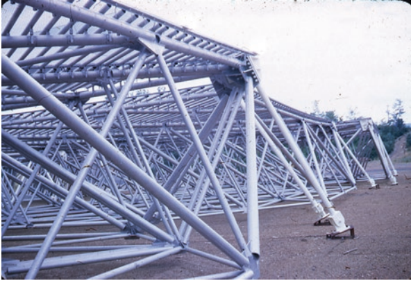
Fig. 9.4 Partially built 600 foot surface backup structures lie on the ground at Sugar Grove in mid-1965. Credit: KIK/NRAO/AUI/NSF
