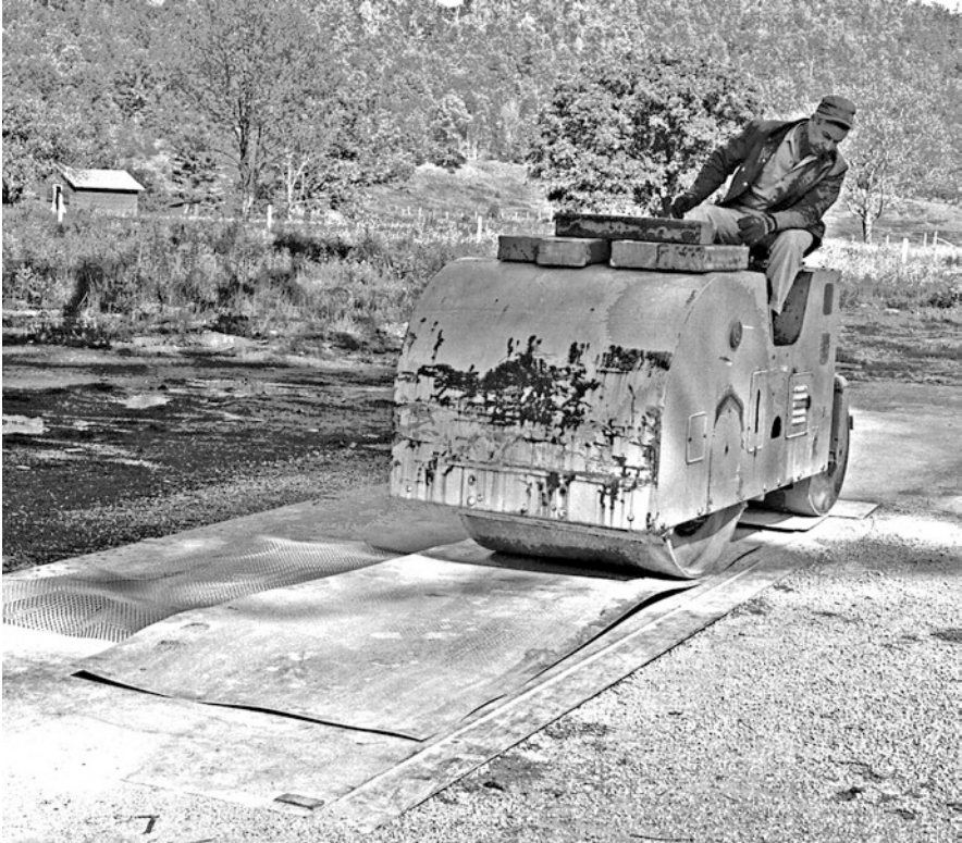
Fig. 4.11 Working in vain effort to smooth the surface of the 300 Foot Telescope, October 1966. Credit: NRAO/AUI/NSF
