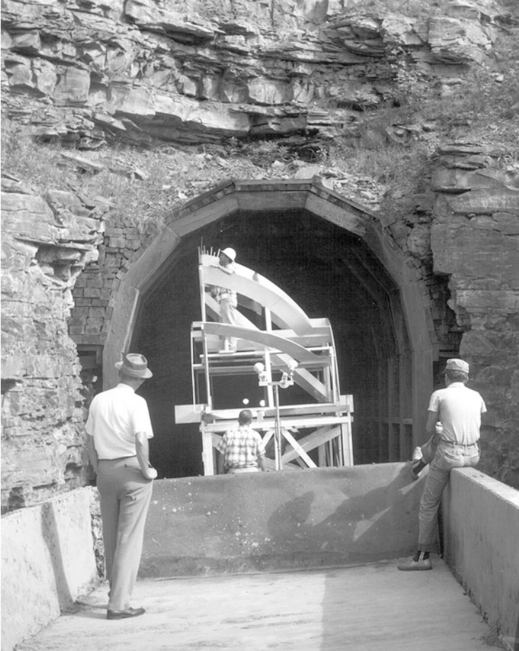
Fig. 4.9 Testing a model of the 17.5 foot spherical bearing for clearance in the rail tunnel through Droop Mountain, 1961. Credit: NRAO/AUI/NSF
