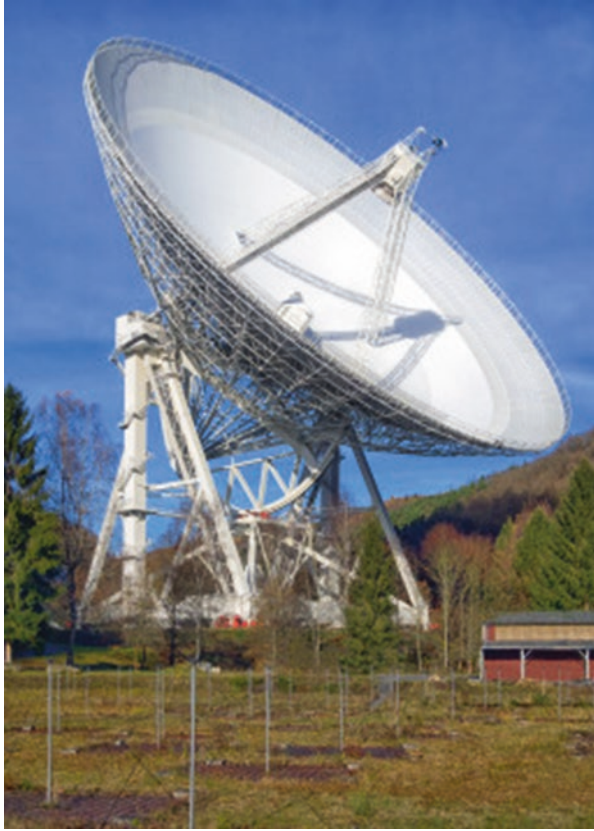
Fig. 9.1 MPIfR 100 meter radio telescope at Effelsberg, Germany designed by Otto Hachenberg. Elements of the International LOFAR Array can be seen in the foreground. Credit: Norbert Tacken, MPIfR
