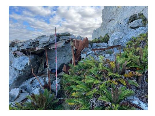
The remains of an Argentine shelter built into boulders on Mount Tumbledown constructed from corrugated metal (repurposed from barrels), angle irons, rocks, timber, and canvas (credit: Falklands War Mapping Project)
