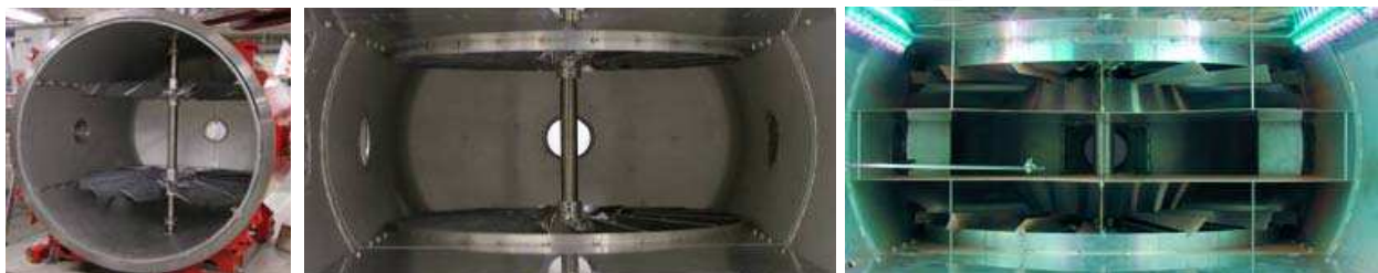
Fig. 6. Photographs into the flow generation section at the AWTS-II facility, Left shows the 1.8m diameter fans installed, Center shows with the upper and lower flow separators and Right the system of vertical and horizontal flow guides compartmentalizing the flow, preventing rotation and excessive turbulence.
