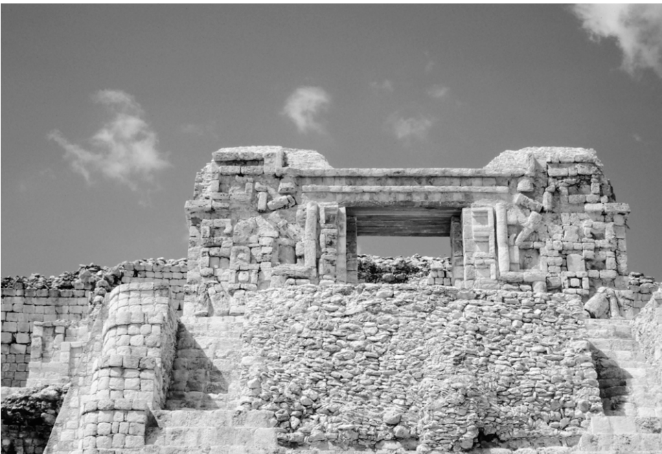
Fig. 27 The restored version shows a cornice which runs along both sides into the remains of the upper ear rings of the monster. There should at least be a distance between the rings and the cornice. Photograph: H. Hohmann 2004
