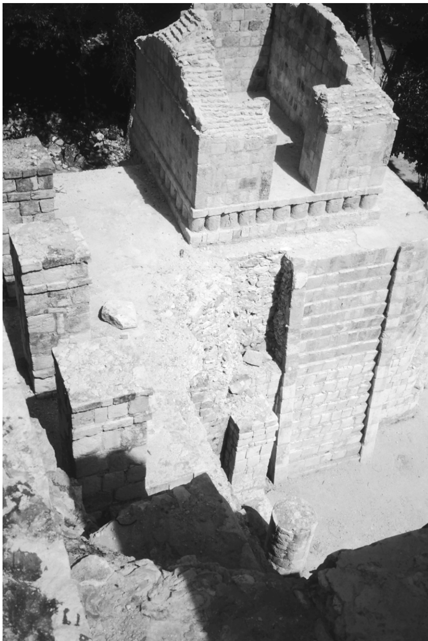
Fig. 95 Room 39 and the southern pseudo Stairway F form the north-eastern temple pyramid. The asymmetry of the position of the stairway is visible. Photograph: A. Drexler 2004
