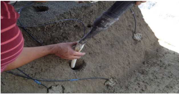
Fig. 4 Backfilling of the top surface of tensiometer location with bentonite slurry
