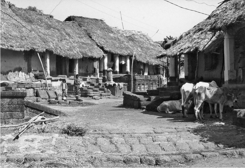
Figure 1.5 Khaṇḍāyata locality: Taḷa Sāhi, Upara Garh in Garh Mantri.
