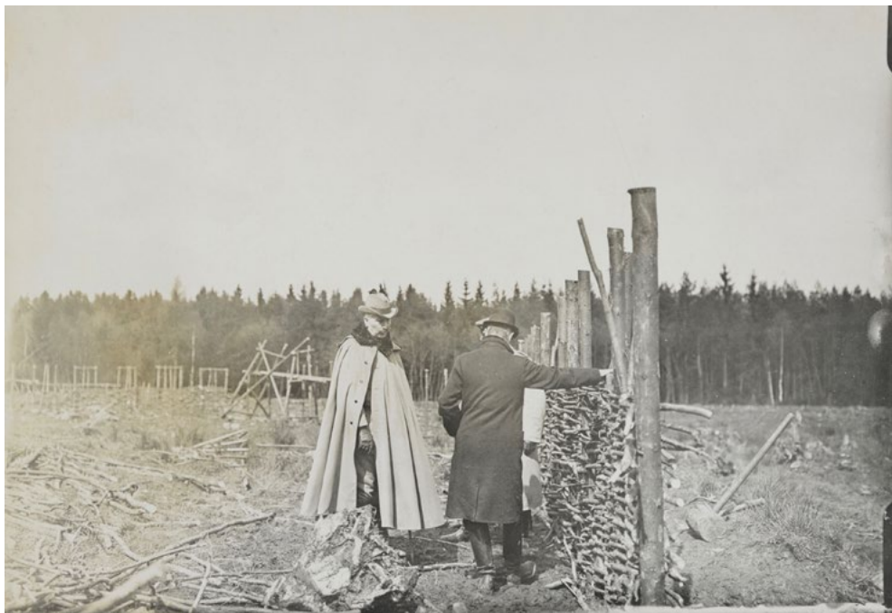
Figure 28.5. Saalburg 1913. Kaiser Wilhelm inspecting work in progress on the wattle-and-daub-construction. Saalburg Archives Neg. No. FA_050.050.009.
