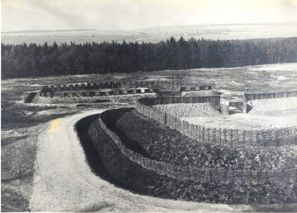
Figure 28.2. Saalburg 1913. Total view of the reconstructed earth works B (foreground) and A. Saalburg Archives Neg. No. FA_050.050.014.
