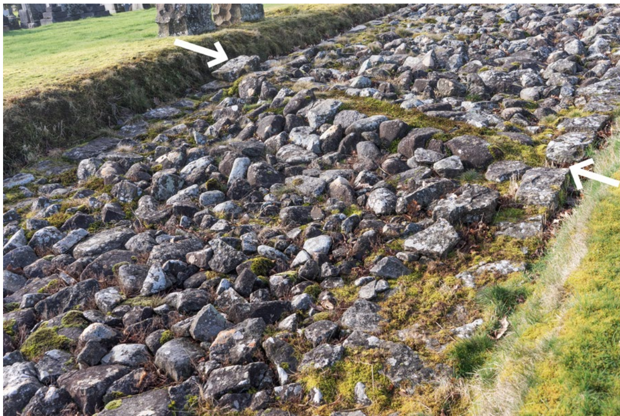
Figure 10.4. Hillfoot cemetery, New Kilpatrick, western part, sector 9. Stone base of Antonine Wall with angular, dressed kerbstones and rubble core. Arrows mark position of stone drain, i.e. the culverts recorded at intervals (© T. Romankiewicz).
