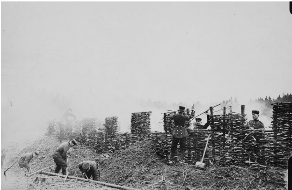
Figure 28.7. Saalburg 1913. Earthwork A with merlons in wattle and daub. Note the rear posts in the middle of each merlon. Saalburg archives Neg. No. FA_050.050.021.
