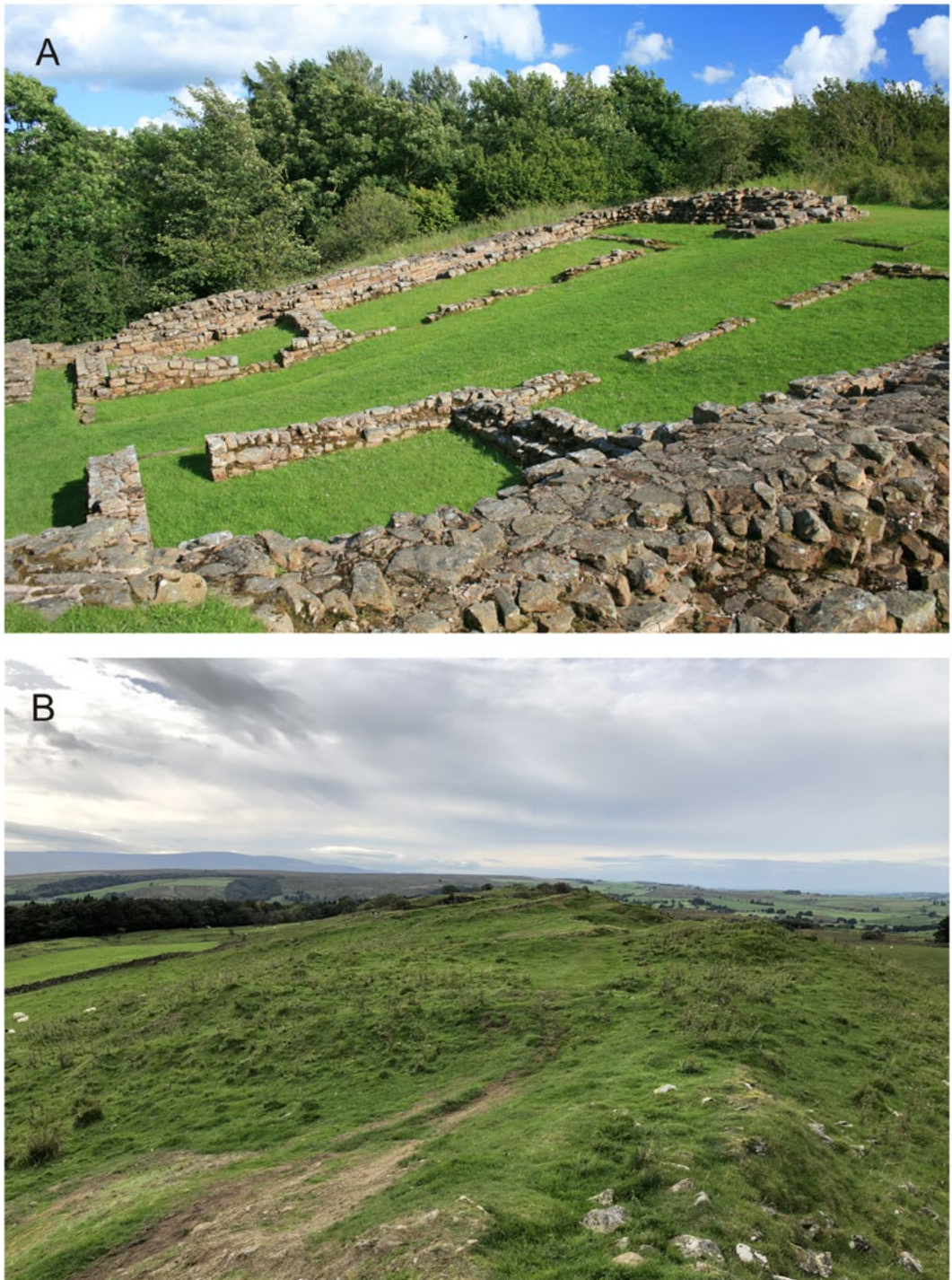
Figure 14.6. A comparison between the plots occupied by milecastle 48 (A) and milecastle 45 (B). While the early Broad Wall milecastle 48 was built on a one-in-five slope, the later – probably Narrow Wall – milecastle 45 potentially contained an artificially-levelled interior.
