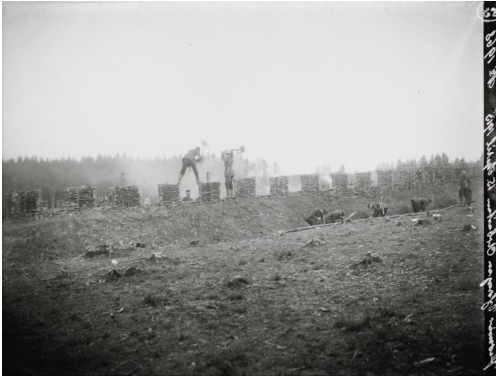
Figure 28.6. Saalburg 1913. Hammering down the posts for merlons. Saalburg archives Neg. No. FG_050.050.014.
