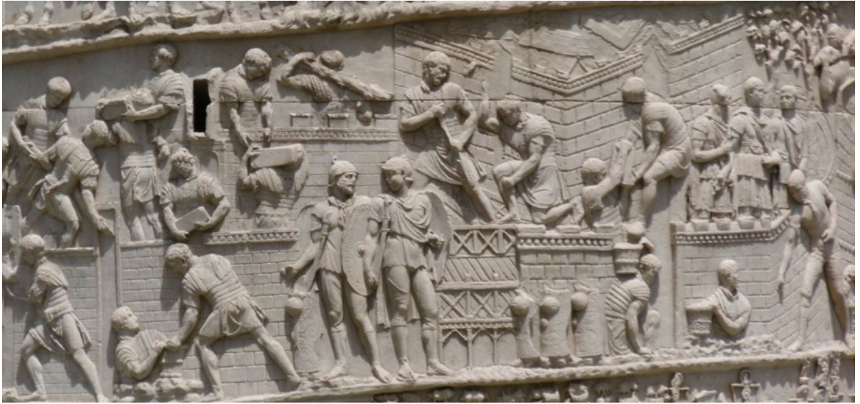
Figure 9.4. Soldiers engaged in construction work. Scenes XI and XII, Trajan's Column, Rome (© Iain Ferris).
