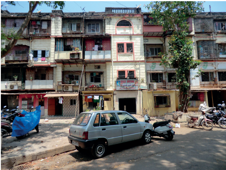
Figure 0.2 One of the BDD Chawls buildings at Delisle Road (N. M. Joshi Marg). © Author.
