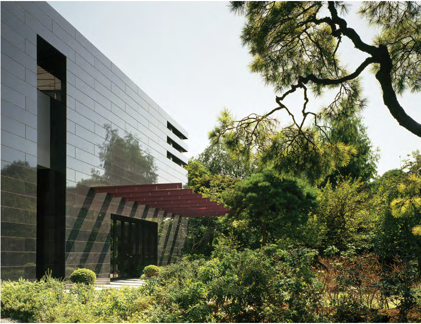
Figure 7.9: Ambassador’s residence, view from garden. Australian embassy, Tokyo, c. 1990.
