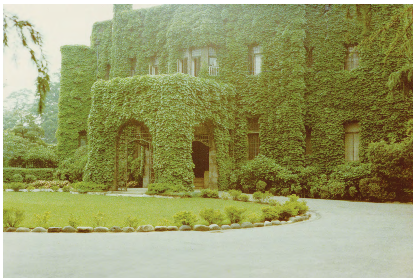
Figure 7.3: Front of the original Hachisuka mansion in Minato-ku, commissioned in 1927 by the Marquis Masaaki Hachisuka (1871–1932) and his grandson, Masauji (1903–1953).
