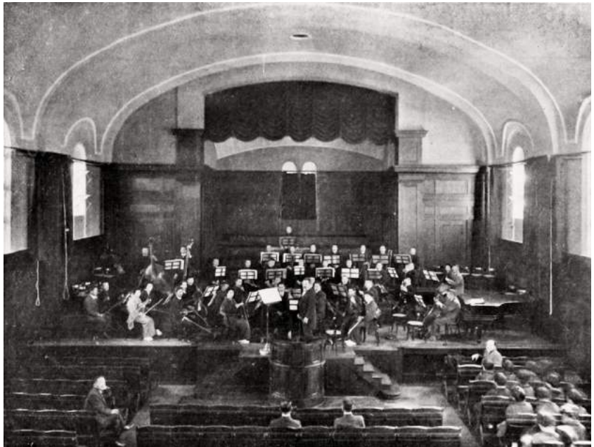
Figure 3.22 Interior of the Nanki auditorium
