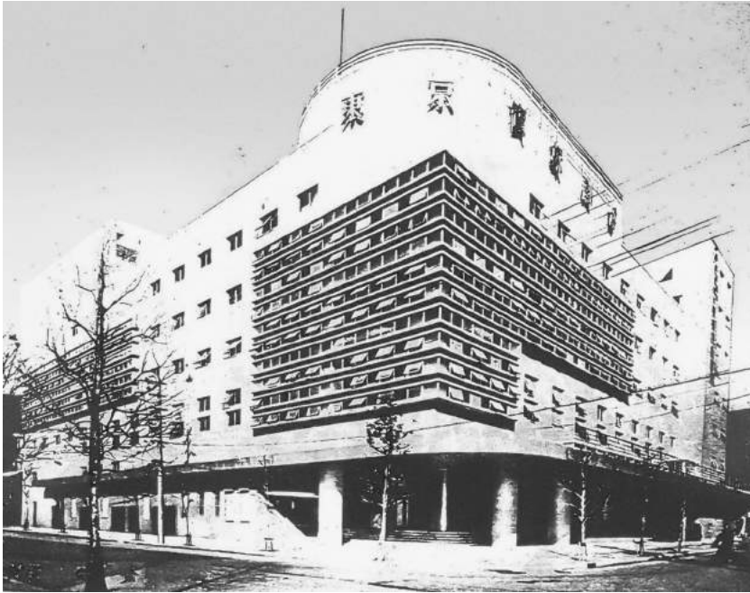
Figure 3.52 Façade of the Tokyo Takarazuka Theatre, located across the street to the north of the Imperial Hotel.
