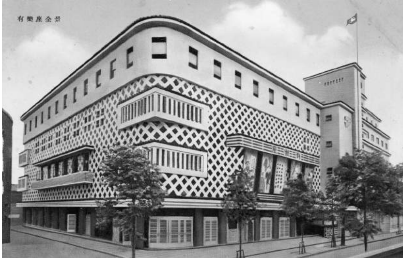
Figure 3.55 Exterior of the Yuraku-za theatre, opened in 1935.
