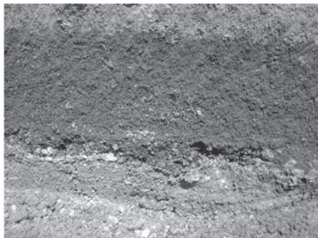
Figure 1. Pavement after milling.
