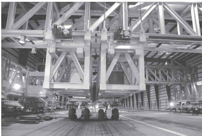
Figure 1. National airport pavement test facility.
