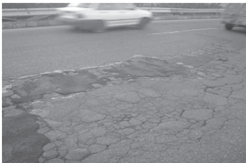
Figure 2. Asphalt distresses.
