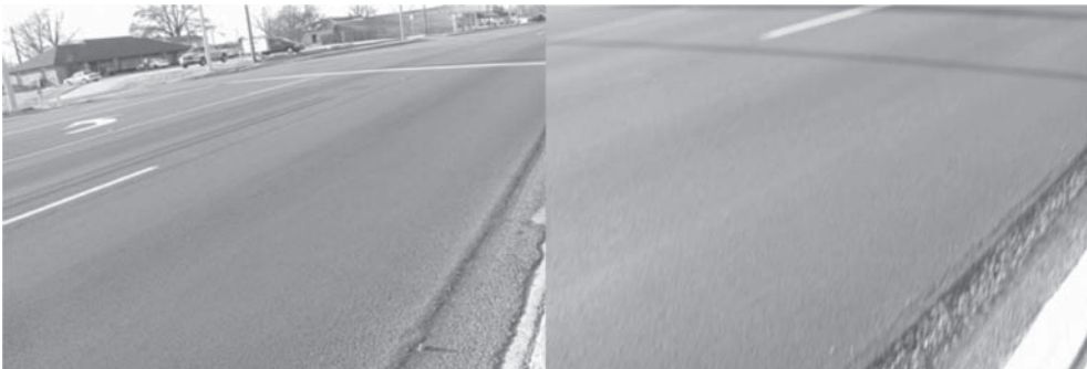
Figure 7. TxDOT type F hybrid overlay mix on US 82 (Texakarna, USA).
