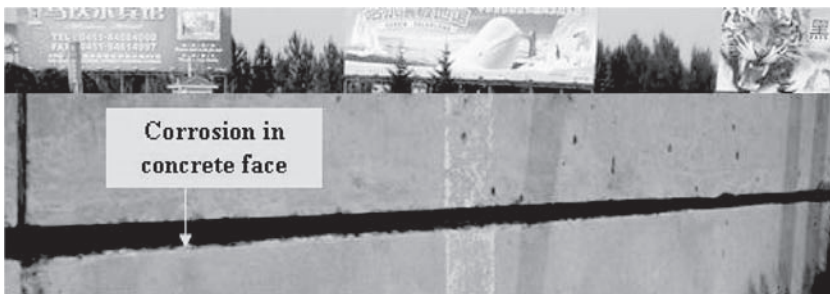
Figure 1. Joint sealant installation section at parking lot in Harbin airport; SJS3 type.
