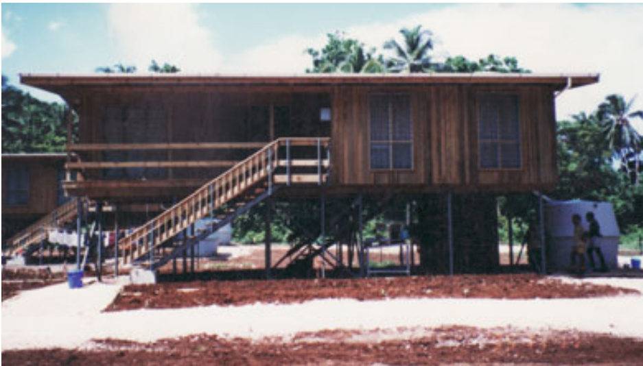
Plate 2-2: Newly constructed relocation house in Putput, 1995.
