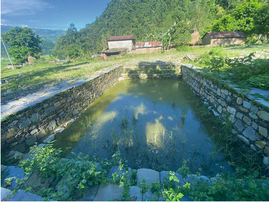
Fig. 4.5 Constructed pond/wetland in WPBP Pokhara (Photo credit: Back to Nature, 2020)
