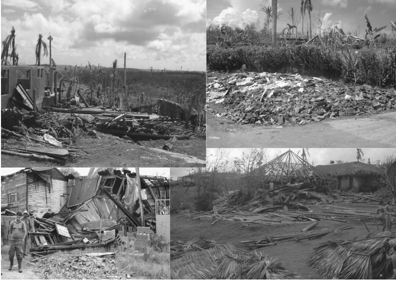
4.2. Photographs showing damage caused by Hurricane Ike in 2008. Clockwise from bottom left: two different modern house designs destroyed by the hurricane, unusable broken house tiles collected for disposal following the hurricane, and one Precolumbian house from the “Taino” heritage village of El Chorro de Maita being rebuilt six days after the hurricane. Photos by (clockwise from bottom left) Roberto Valcárcel Rojas, Roberto Valcárcel Rojas, Jago Cooper, and Jago Cooper.
