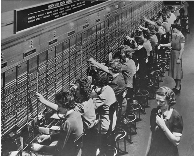
FIGURE 2.1 An example of circuit switching: telephone operators at “Central” using a plug board to connect phone calls.
