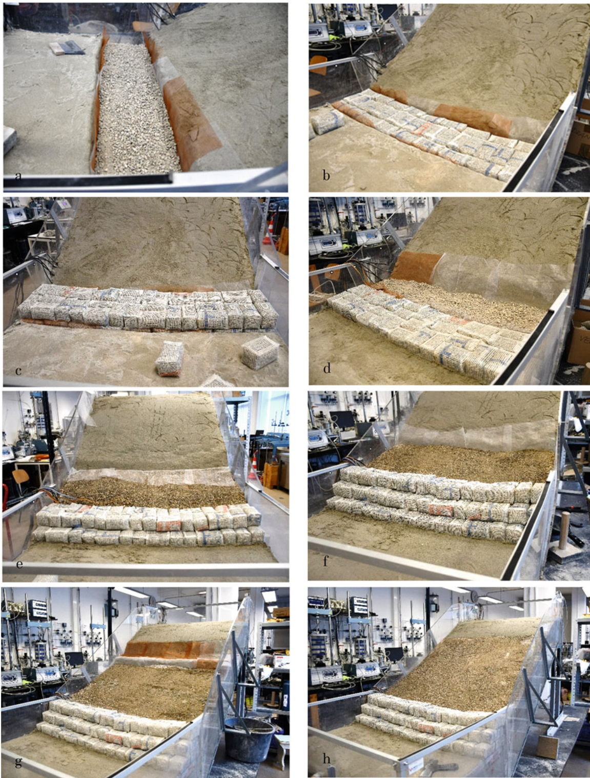
Fig. 9 Installation of the gabion wall and buttressing embankment behind the wall in a prepared silty slope: (a) excavated foundation pit with compacted layer of gravel, (b) first row of gabion boxes installed in foundation pit, (c) second row of gabion boxes installed, (d) filled buttressing embankment behind the gravity wall separated from the
