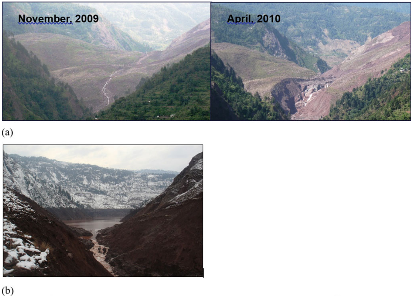
Fig. 8 (a) Front view of Hattian landslide dam, before and after failure, (b) Front view of the dam immediately after breaching (Konagai and Sattar 2011)
