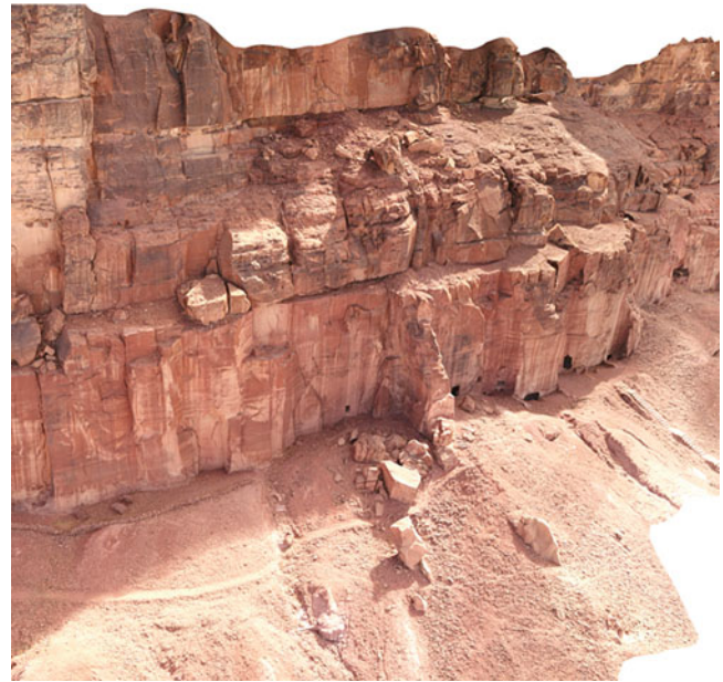
Fig. 21 Collapsed blocks at the toe of the cliff with the pedestrian pathway passing through. This is a clear example of a pathway standing too close to the cliff and exposing visitors to a potential risk of being involved in a rockfall
