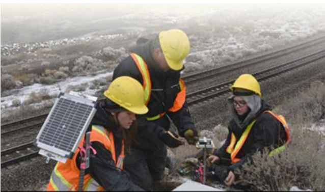
Fig. A.5 The GSC conducts geohazard studies to reduce risks to people and infrastructure, here installing equipment to monitor landslide activity above a critical railway corridor in central BC
