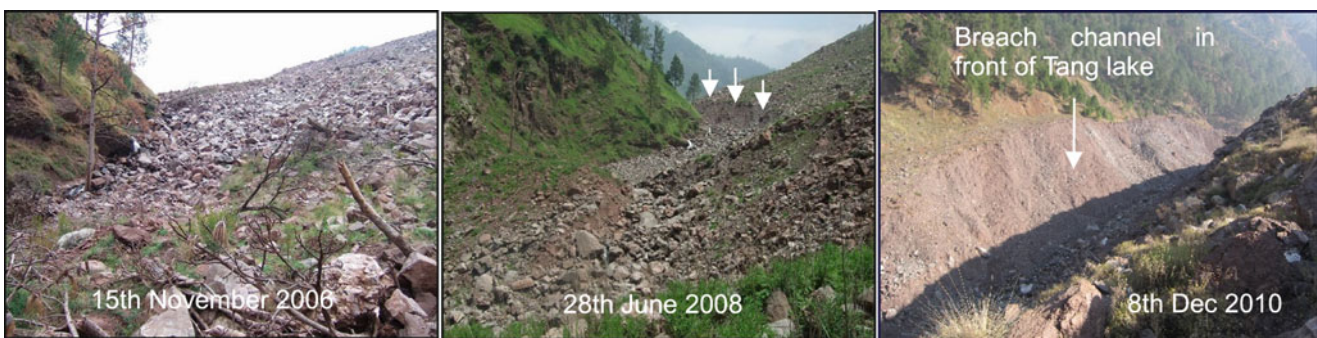
Fig. 6 View of the path of water flowing from the Tang Lake. The surface change can be observed between November 2006 (left) and June 2008 (middle). While the right most figure shows the breach channel
