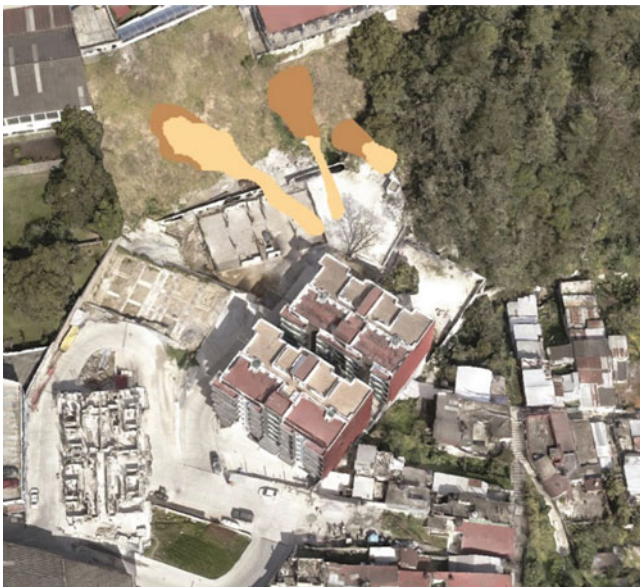
Fig. 10 New buildings constructed in areas highly susceptible to landslides in the Juárez neighborhood, 2023
