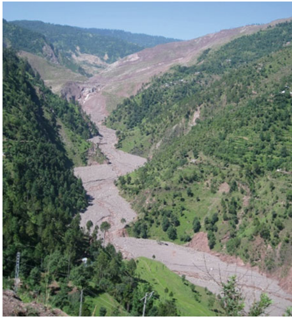
Fig. 9 Partially breached Hattian dam and debris deposit along the Karli River. (Photo taken on sixth June 2010 at N 34.156567°, E 73.744833°)
