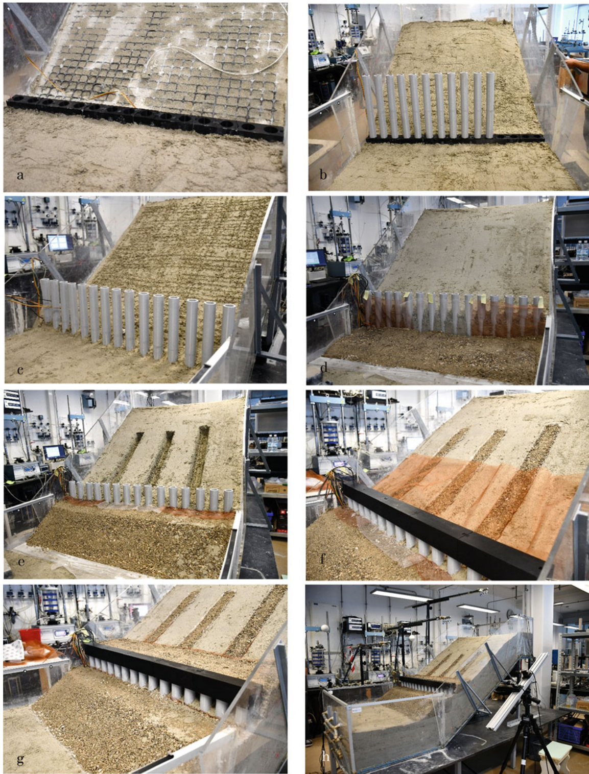
Fig. 10 Installation of pile wall construction and buttressing counterfort in the front of the wall in clayey slope: (a) setting and fixing foundation beam to the model base, (b) installation of piles in foundation beam, (c) built in the soil layers in the slope, (d) base of buttressing
