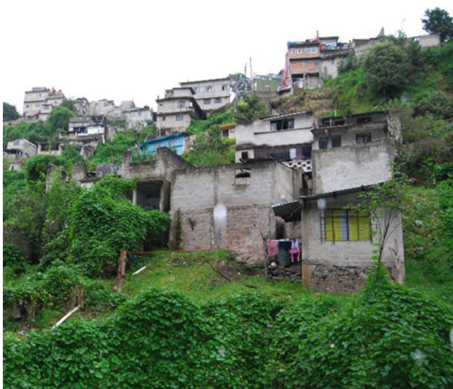
Fig. 6 Housing continues to be built, moving toward the bottom of the ravines, lacking proper drainage systems
