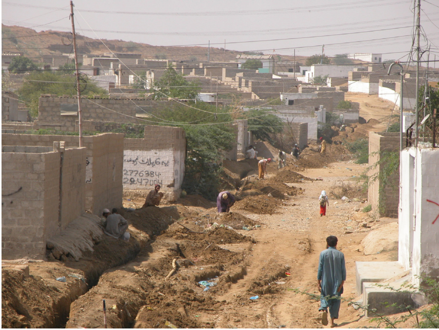
FIGURE 8.3. Orangi Pilot Project self-help wastewater sewerage and community development. Photo courtesy James Wescoat.
