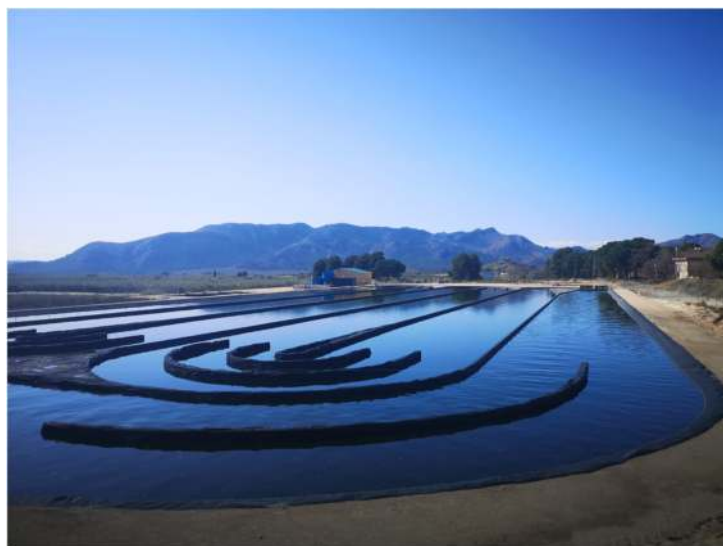
Figure 5.2 Image of raceway reactors utilized for wastewater treatment at Agramon (Spain) designed and operated by Aqualia.
