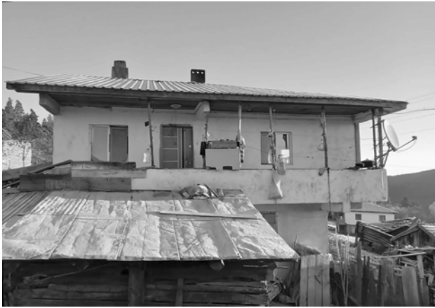
Figure 7.3: West façade of the dwelling with a metal door salvaged from Istanbul
