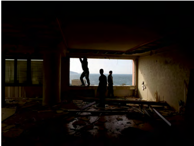
Figure 5.3: Salvaging an apartment building in Kadıköy 6
