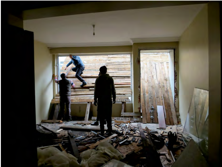
Figure 5.6: Installing the debris slide 9
