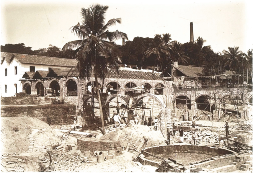
Figure 3: Mangalore Tile-Works at New Jeppu under Construction. Unknown. QU-30.016.0073. BMArchives.
