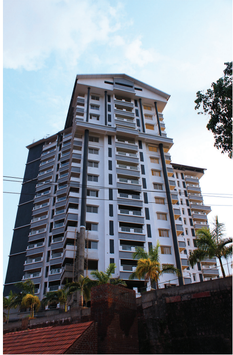
Figure 9: From behind the tile works, the future.
