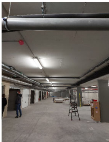
Figure 8. Views on the transfer slab with 10 mm of fire protection added.
