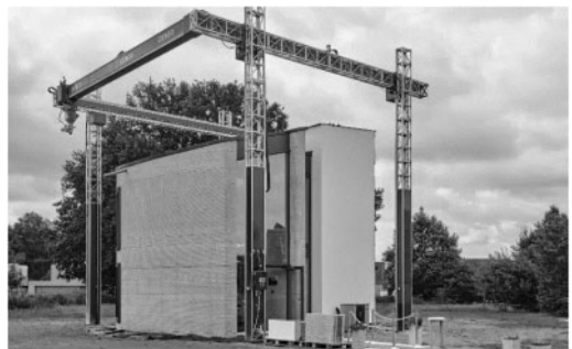
Figure 1. The 3D printed house at KampC – Oevel, Belgium.
