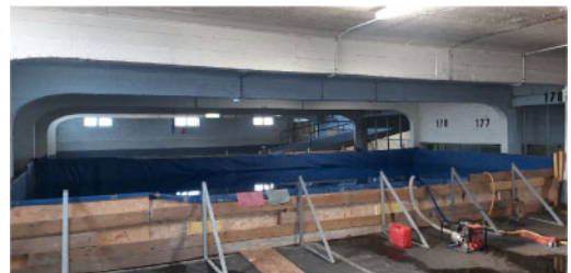
Figure 7. Load test existing parking building.
