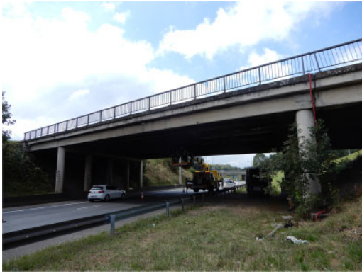
Figure 1. Global photo of the bridge.
