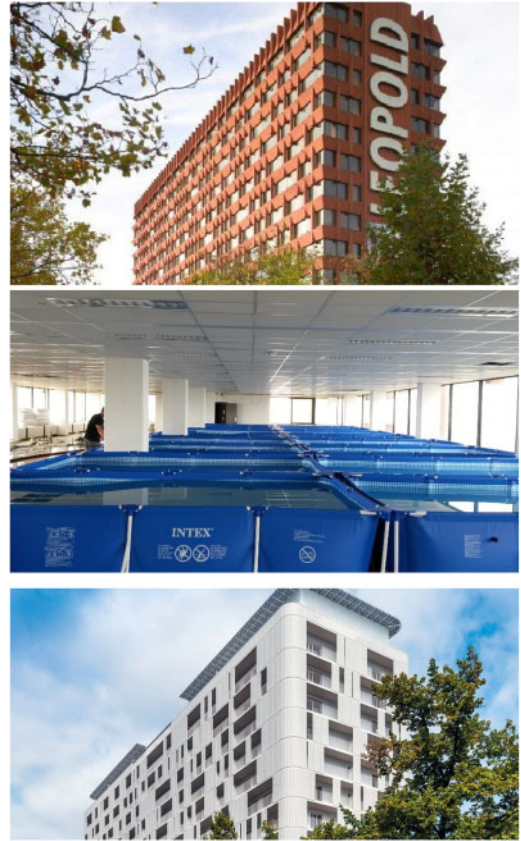
Figure 6. Building before, during load test and after rehabilitation.
