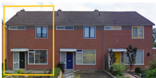
Figure 1. The building assessed: the modelled end unit is identified via a yellow rectangle.
