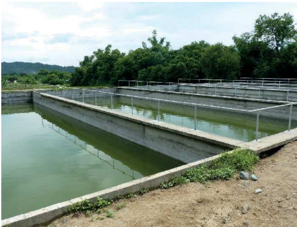
Figure 11.8 Starting up period of faecal sludge lagoon system, San Fernando City, Philippines. In this case, lagoon basins were seeded with activated sludge from a nearby wastewater treatment plant (photo: David M. Robbins).
