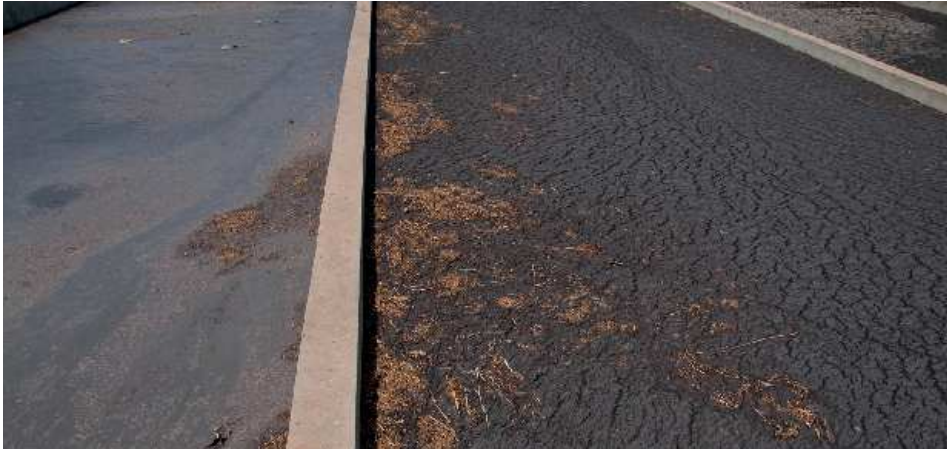
Figure 7.2 Freshly loaded and partially dewatered faecal sludge on unplanted drying beds at Niayes faecal sludge treatment plant, Dakar, Senegal (photo: Linda Strande).
