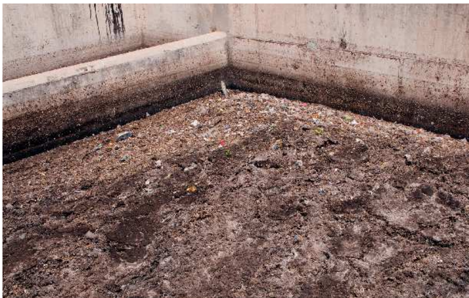
Figure 3.2 Settling tank at Niayes faecal sludge treatment plant in Dakar, Senegal (photo: Linda Strande).
