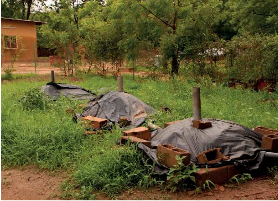
Figure 3.9 Biogas reactors at 2iE in Ouagadougou, Burkina Faso (photo: Linda Strande).
