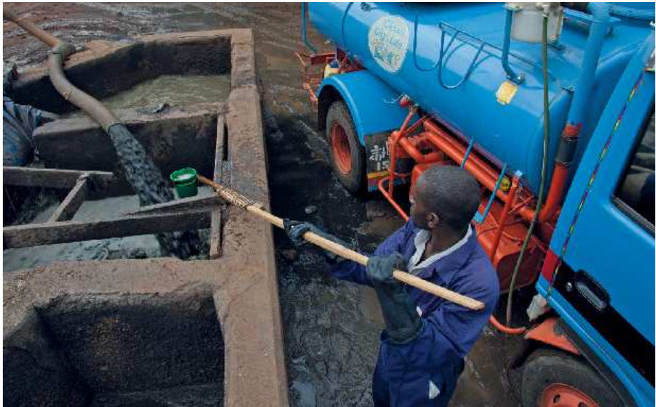
Figure 18.3 Implementation of the FAQ method (Faecal Sludge Quantification and Characterisation) in Kamapla, Uganda (photo: Lars Schoebitz).
