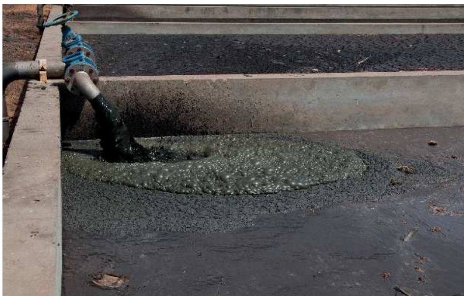
Figure 7.4 Loading of the beds at Niayes faecal sludge treatment plant, Dakar, Senegal (photo: Linda Strande).
