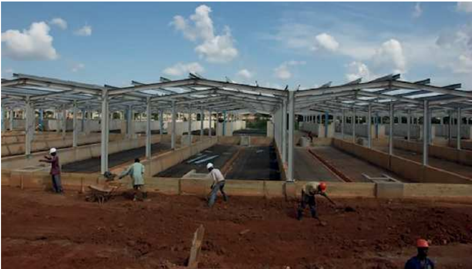
Figure 18.1 Drying beds for faecal sludge treatment under construction at Lubigi faecal sludge treatment plant in Kampala as part of the Lake Victoria Protection Stage I Project funded by KfW, EU and Government of Uganda/NWSC (photo: Lars Schoebitz).
