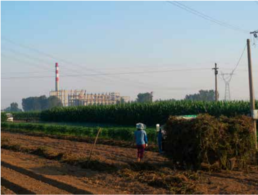
Figure 4.1 Construction site of Panguanying incinerator, July 2013
