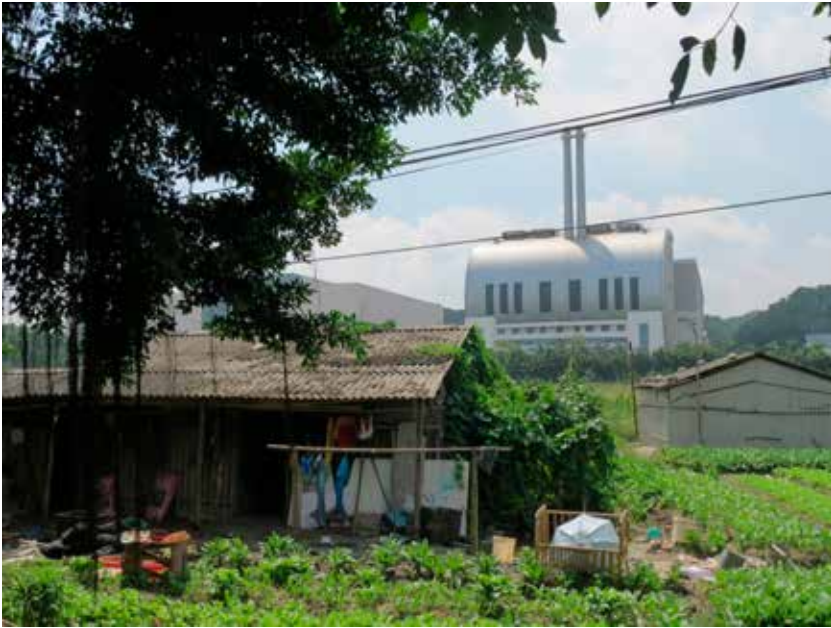
Figure 2.1 Guangzhou Likeng incinerator, July 2013
