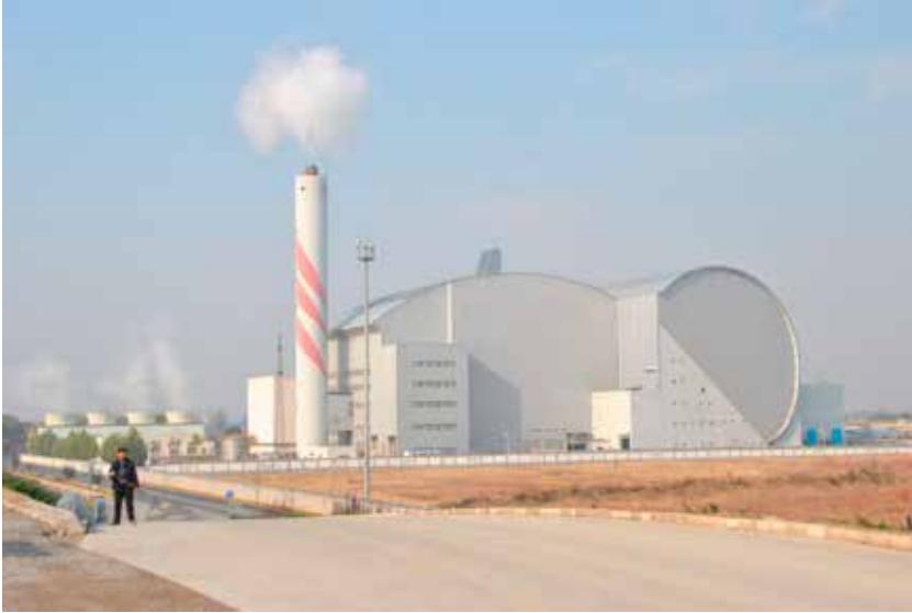
Figure 3.1 Gaoantun incinerator, November 2012
