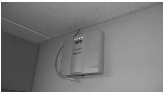
**Figure 9.3** Example of poor cable installation.
