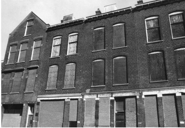
Vacant houses closed with bricks in Bospolder-Tussendijken
