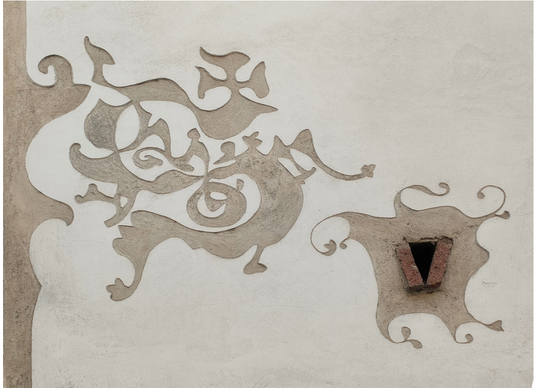
Fig. 8. Details of the façade: sgraffito emblem. Photographs by the authors.
