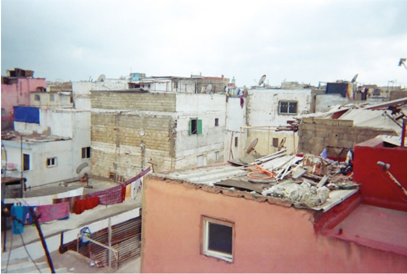
Figure 2: Rooftop view of the appropriated grid.
