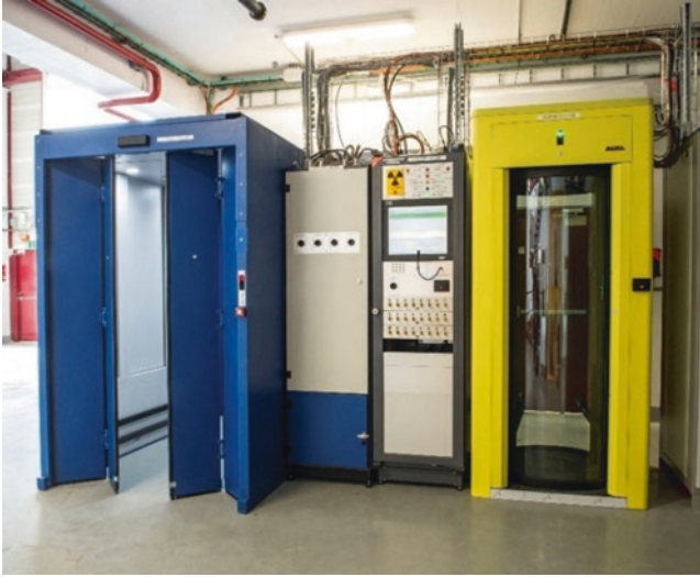
Fig. 5.4 Access doors of the Proton Synchrotron at CERN. Right, a personal door, letting only one authorized person pass at a time. Left, a material lock, in which the two doors cannot be open at the same time. Centre, the access control system with interlock key panel. (Photo: CERN)
