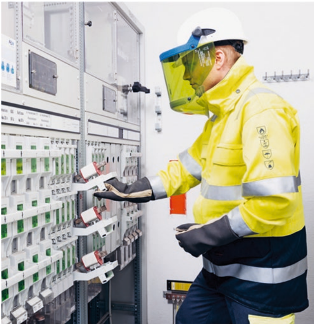
Fig. 4.2 Electrician equipped with PPE: Helmet, arc-flash resistant visor, insulating gloves, fire-resistant jacket. Not visible: shoes with isolating soles. (Image credit: SUVA)
