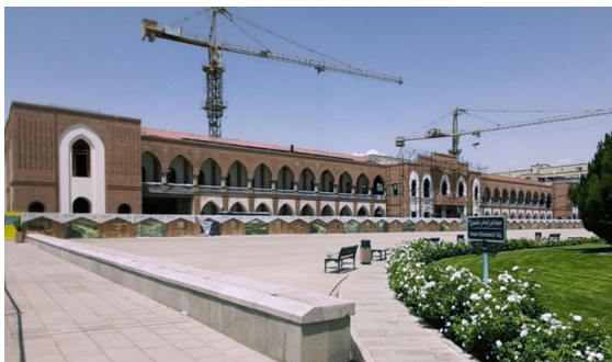
Figure 53: The ongoing reconstruction project of the Baladiyeh
