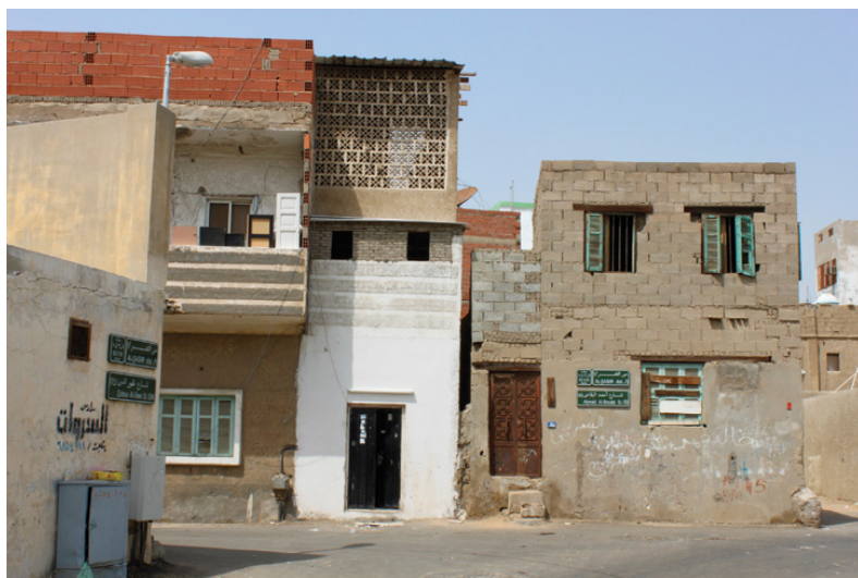
Figure 3.4 Small residential units constructed on an ad hoc basis in al-Thaghr district. Photo: © Stefan Maneval 2010.
