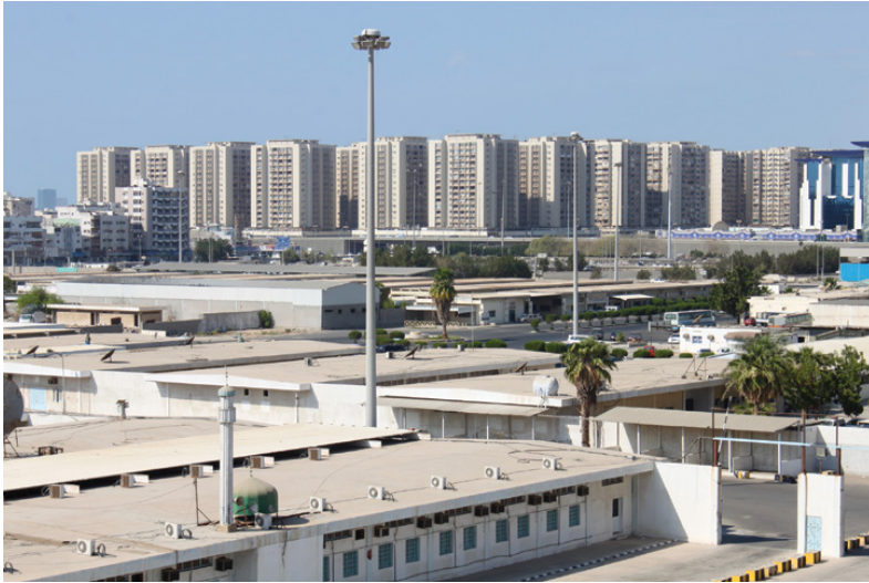
Figure 6.4 The Jeddah Rush Housing Project. In the foreground: facilities of the pilgrims' city at the old airport. Photo: © Stefan Maneval 2012.
