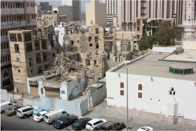
Figure 1.8 Ruin of an old residential building in al-Balad, 2012. Photo: © Stefan Maneval.
