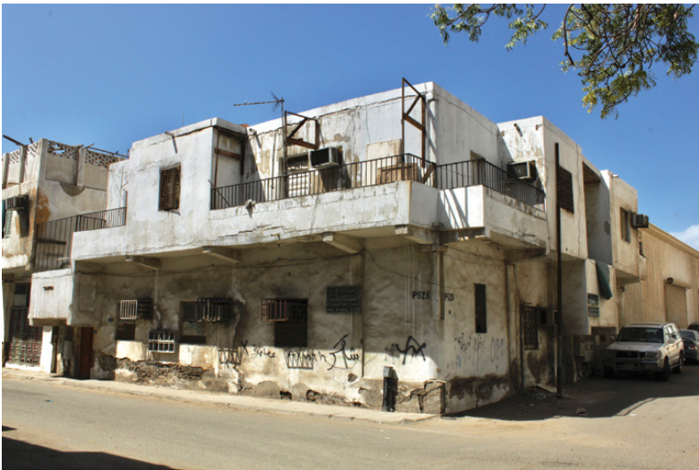
Figure 3.2 Concrete building, constructed around 1960, in al-Hindāwiyya. Photo: © Stefan Maneval 2011.
