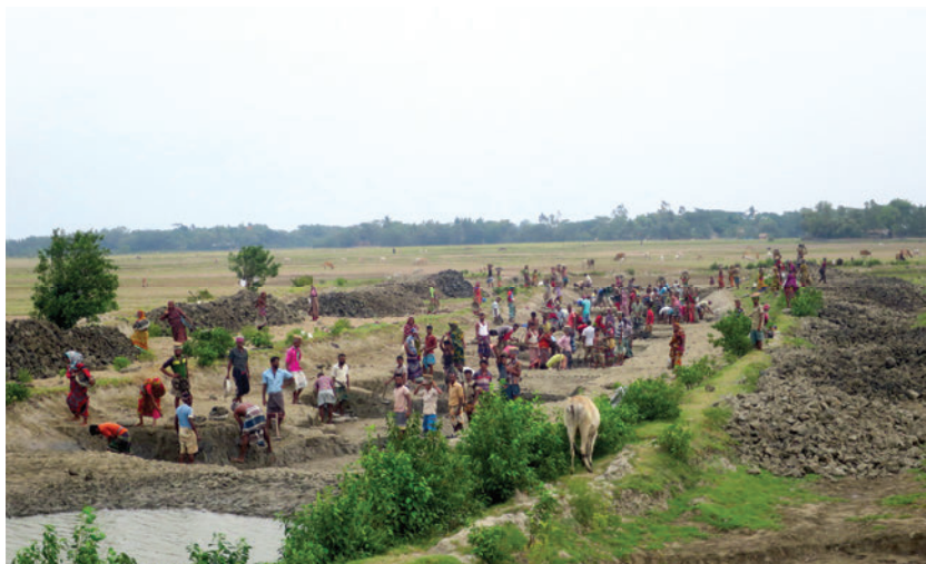
FIGURE 2.2. Canal excavation in Nodi, May 2015. Photo by author.
