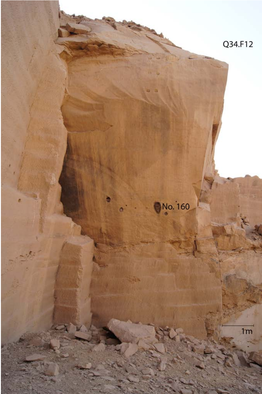
NO. 160 Quarry 34, east-facing (F12)
