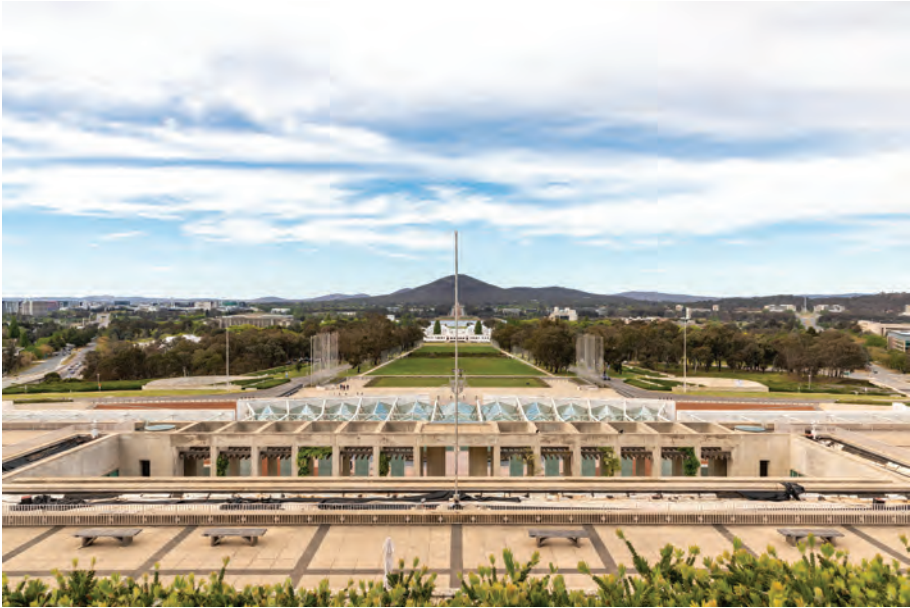
Figure 1.7 The parliament houses of Canberra, the new house in the foreground, looking towards the old house in the background. © Dietmar Rabich, 20 October 2019. ‘Canberra (AU), Parliament House and Old Parliament House – 2019 – 1767’. Source: Wikimedia Commons, reproduced on the basis of a CC BY-SA 4.0 licence. Available at: https://commons.wikimedia.org/wiki/File:Canberra_(AU),_Parliament_House_and_Old_Parliament_House_-_2019_-_1767.jpg (accessed 6 December 2022)
