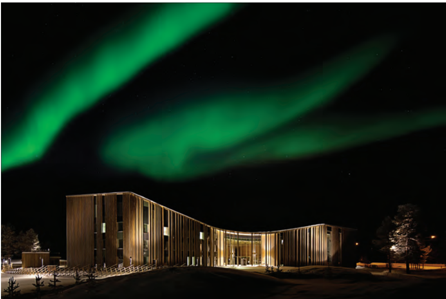
Figure 25.1 HALO Architects, Sajos, Inari, 2012. Exterior view, south elevation (photograph by Mika Huisman, 2012). © Decopic Oy
