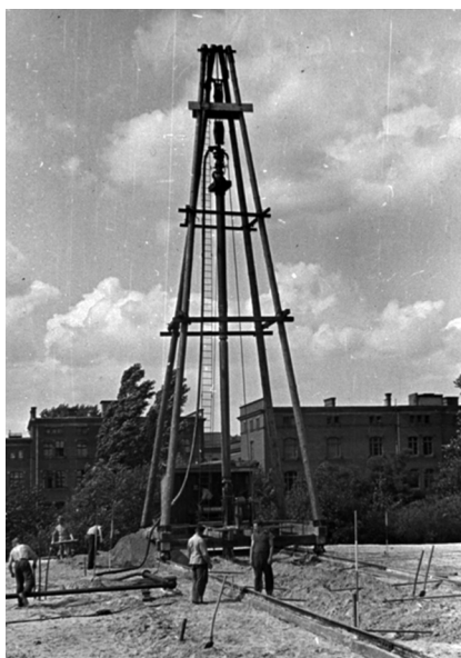
Figure 2.7 Vibro compaction employing wooden gantry, 1939. (Courtesy of Degebo, Berlin, Germany.)
