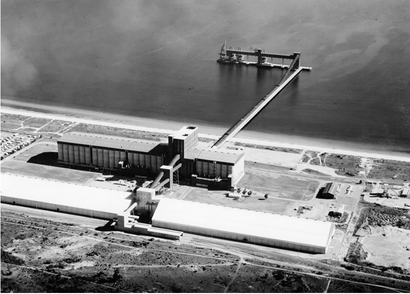
Figure 2.16 Areal view of the Grain Terminal at Kwinana, Western Australia. (Courtesy of Keller Group plc, London, UK.)
