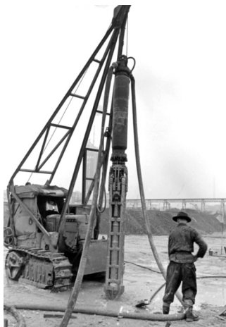
Figure 2.18 First generation vibrocats, 1956. (Courtesy of Keller Group plc, London, UK.)
