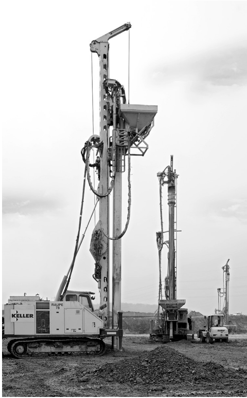
Figure 4.2 Vibrocat with bottom feed vibrator. (Courtesy of Keller Group plc, London, UK.)
