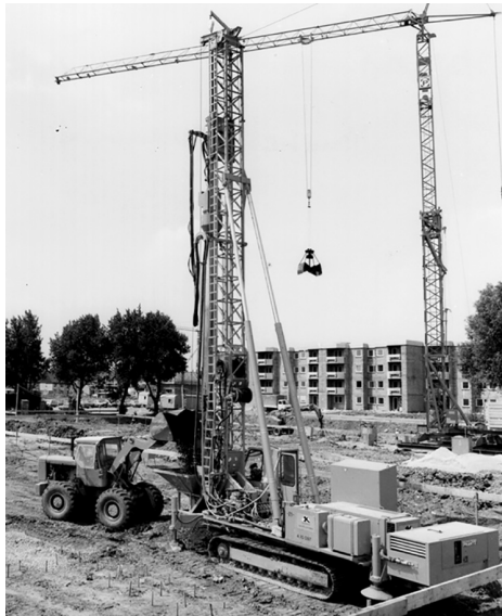
Figure 2.19 Vibrocat developing downward thrust, 1977. (Courtesy of Keller Group plc, London, UK.)
