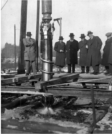
Figure 2.4 Trial compaction at Berlin. (Courtesy of Degebo, Berlin, Germany.)
