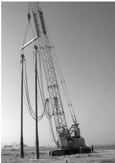
Figure 3.41 Vibro compaction equipment set up for S700 twin vibrator operation. (Courtesy of Keller Group plc, London, UK.)
